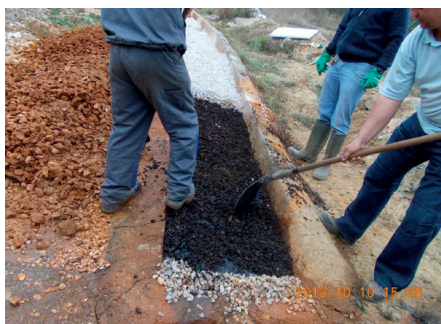
Fig. 10 Installing the passive AMD treatment channel
