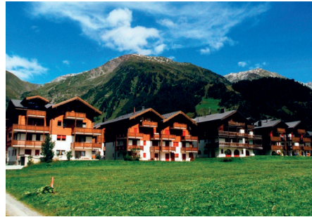
Fig. 5 Oberwald/VS – A distributor network at the western portal of the Furka Rail Tunnel conducts the tunnel water to the heat pumps for each consumer. Tunnel water temperature: 16 °C, thermal capacity: 960 kW (Photo: J. Wilhelm, Pully)
