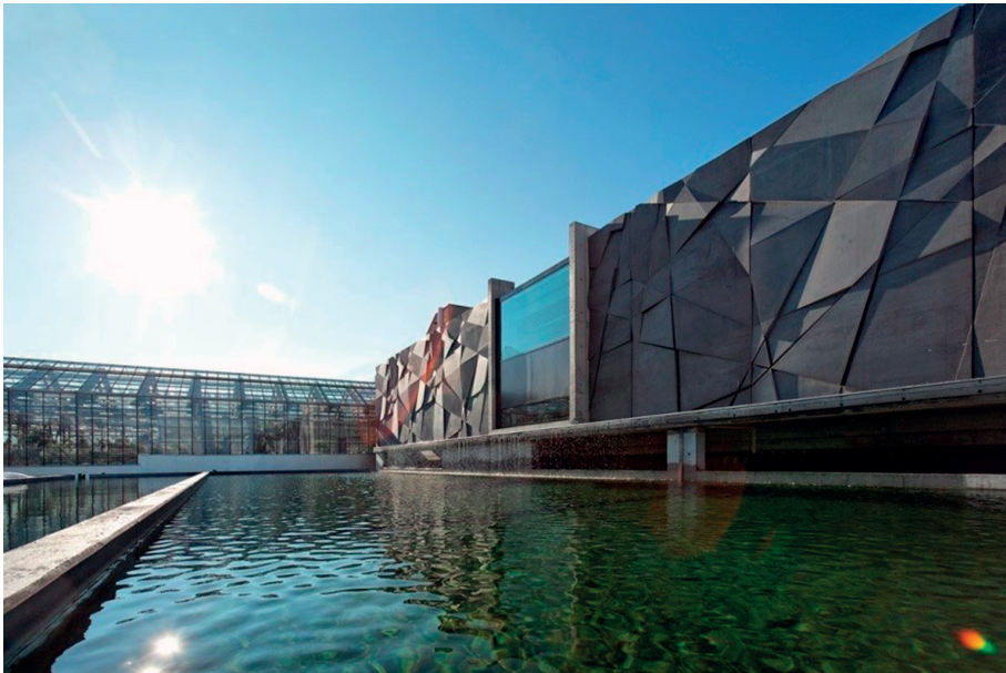
Fig. 7 Warm drainage water from the Loetschberg Base Tunnel (160 l/s, 17 °C) is used as the energy base. Fish such as sturgeon and perch, which thrive in warm water, are raised in the Tropenhaus Frutigen fish hatchery basins (in front) as well as tropical fruits are grown in greenhouses (in the back)
