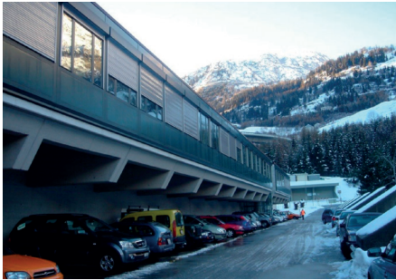
Fig. 4 Airolo/TI – The Entertainment Centre of the Gotthard Road Tunnel at the southern portal has been heated and cooled geothermally since 1979. Tunnel water temperature: 17 °C, thermal capacity with 4 heat pumps: 720 kW (Photo: Geowatt AG, Zurich)
