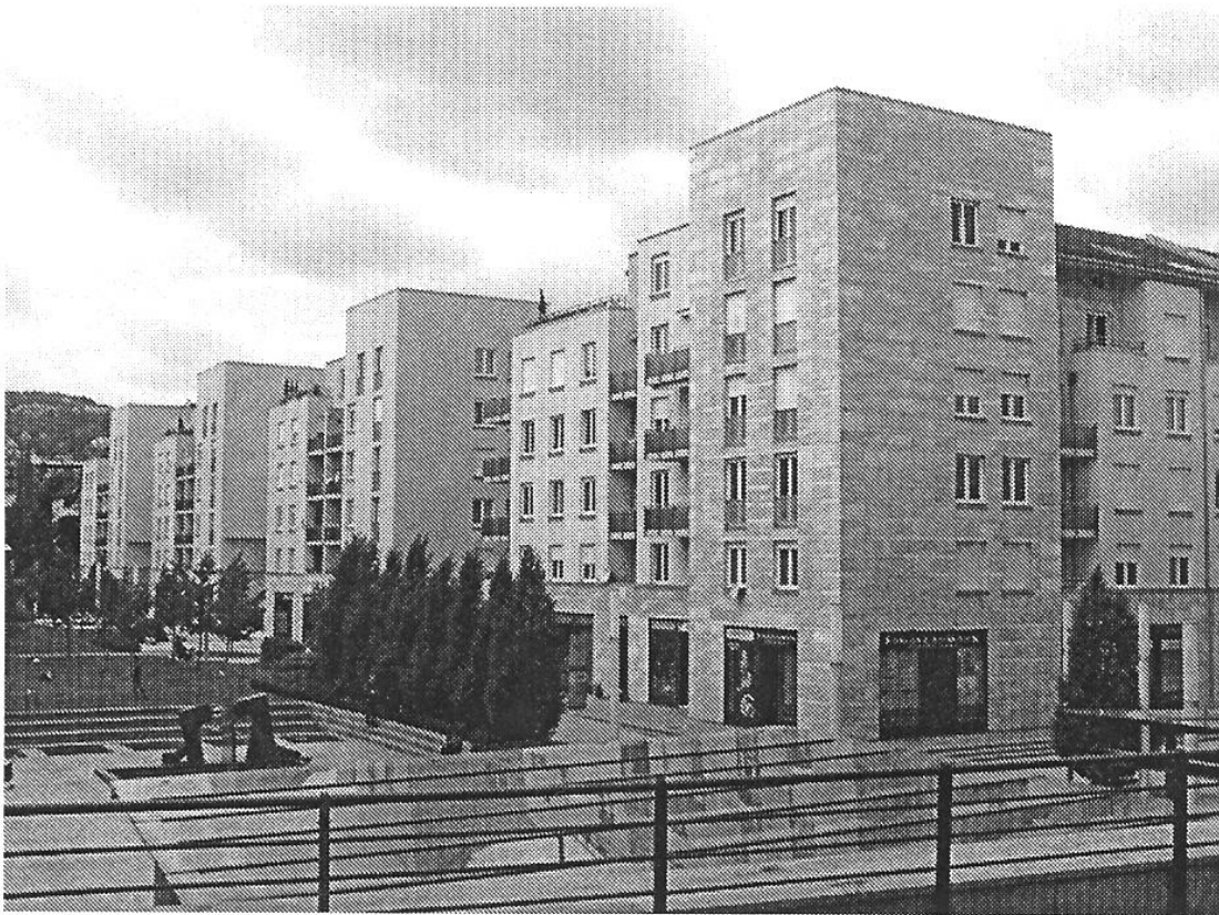
Fig. 8.11 The MOM residential park. This prestigious development was built on the site of a former optical factory in 2002
