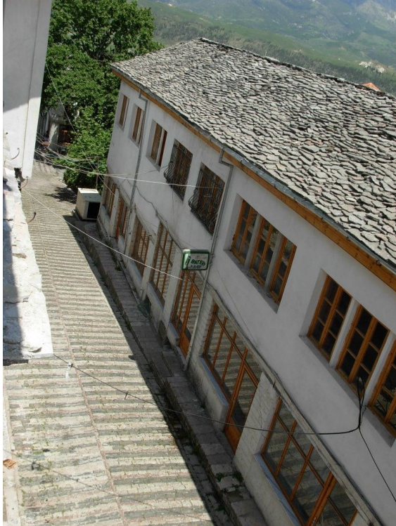
Figure 5. Part of restored bazar area, Gjirokastra (Photo: Bosse Lagerqvist)
