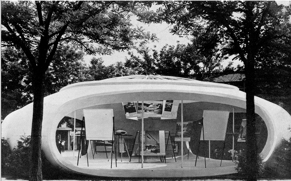
Fig. 1. Shaped dwelling of sprayed concrete designed by John Johansen - US display model at Zagreb International Trade Fair 1956
