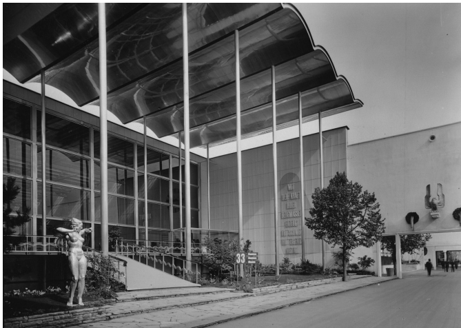
Fig. 10. Aluminium Pavilion, Architect Jos. Schütz, BSA Zurich, Photographer Louis Beringer, 1939
