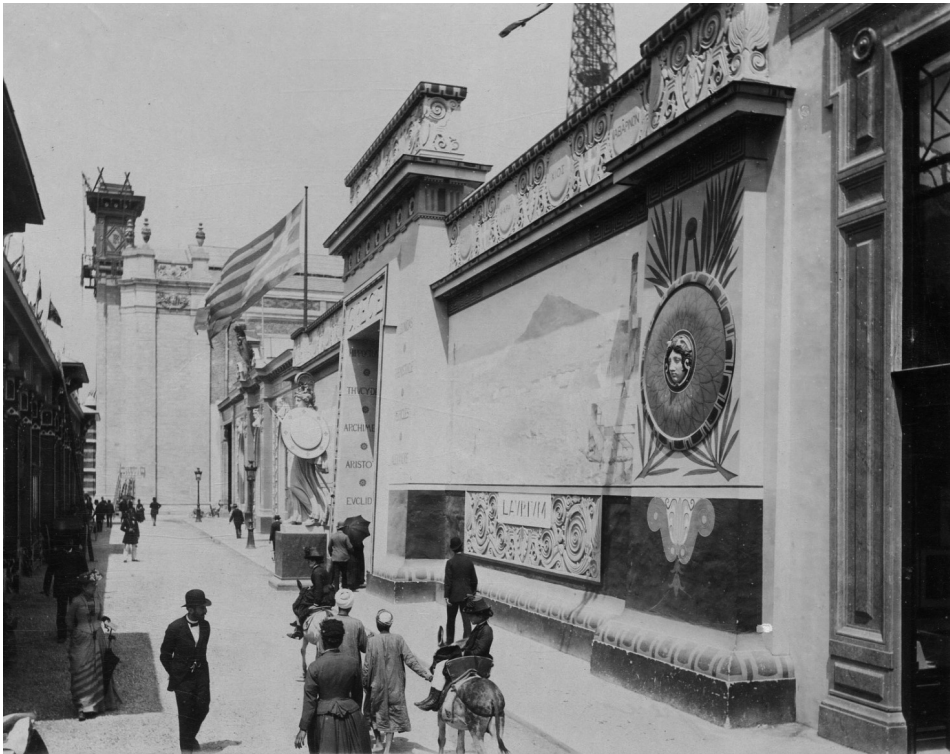
Fig. 8. View of the Greek Pavilion, Paris, 1889
