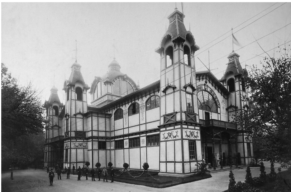
Fig. 4. Croatian Industry, Crafts, Education, Ethnography and Economy Pavilion, architect Vjekoslav Heinzel, photo made by György Klösz, 1896
