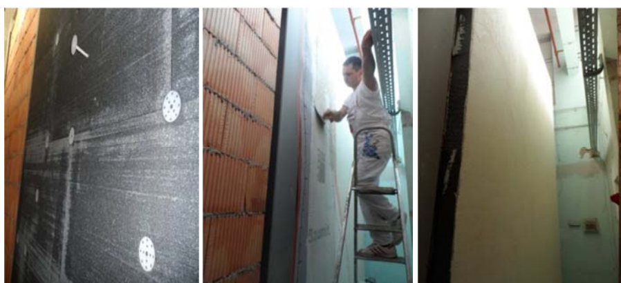
Fig. 10. Construction process of infill specimen MW2
