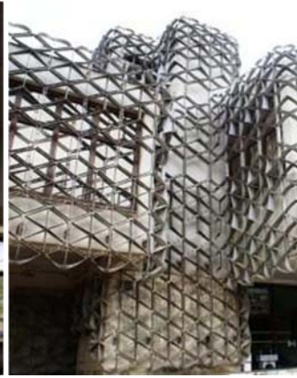
Fig. 5. Metal grid covering the façade (photo: Eris Kajtazi)
