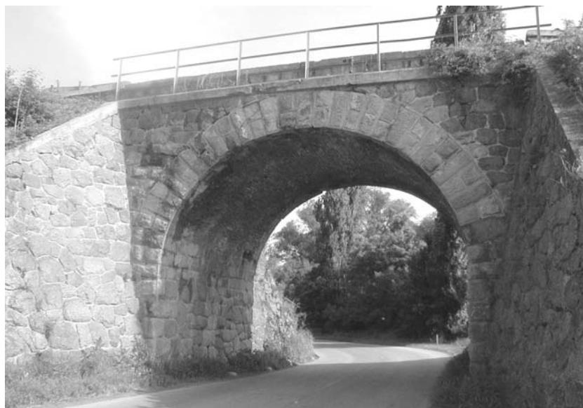
Fig. 1. Typical single span railway masonry arch bridge in Hungary
