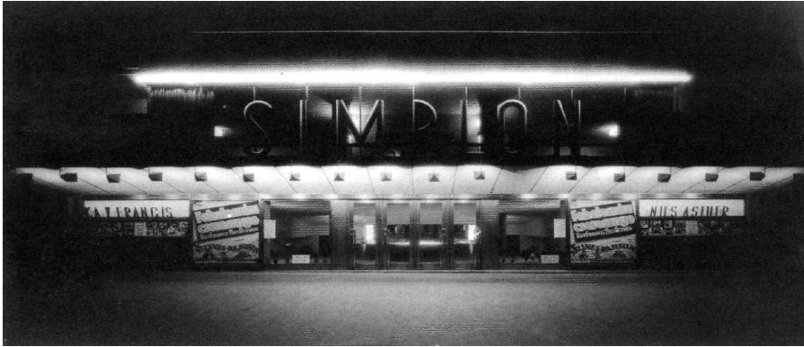
Fig. 1. Simplon Apartment Building and Movie Theater, built in 1934
