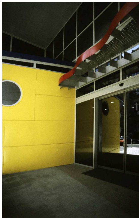
Fig. 9. Corner of the main entrance
