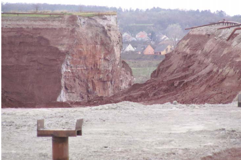
Fig. 1 The collapsed dam
