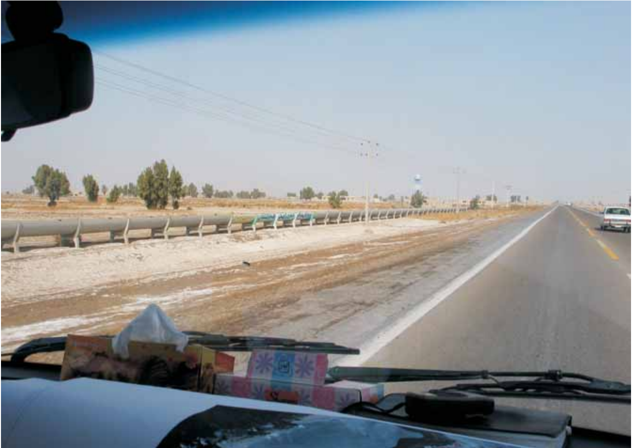
Modern irrigation canal
