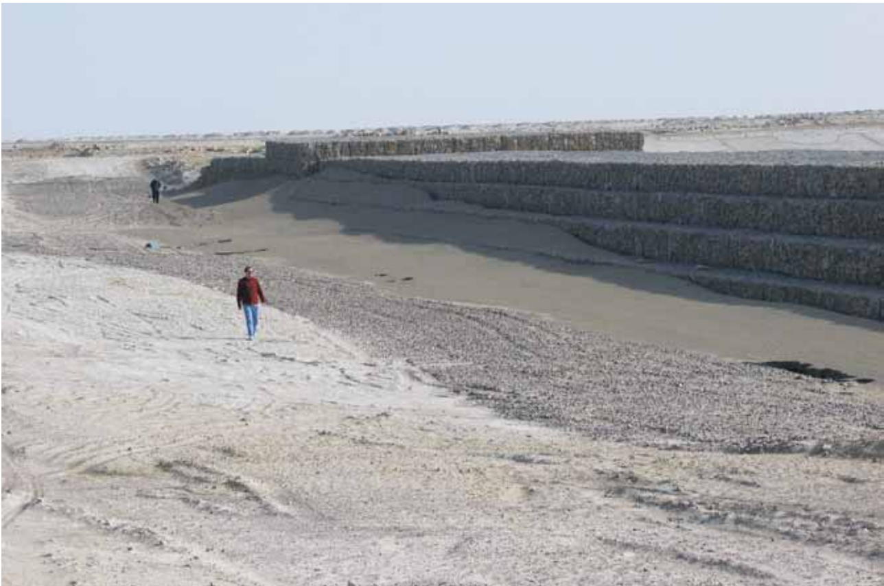
Control structure at the outflow of Hamoon Hirmand
