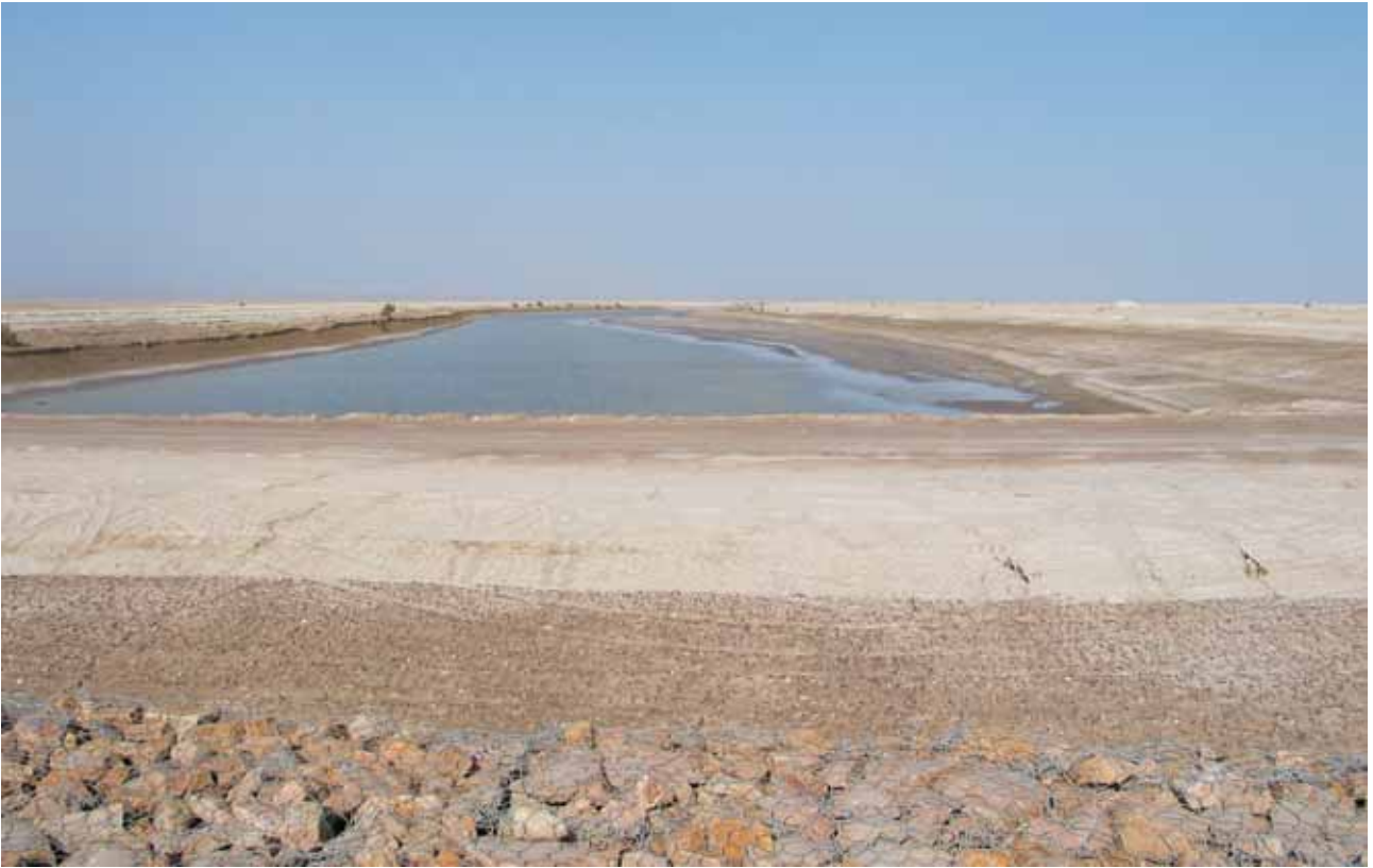
View from the control structure of the overspill canal of Hamoon Hirmand
