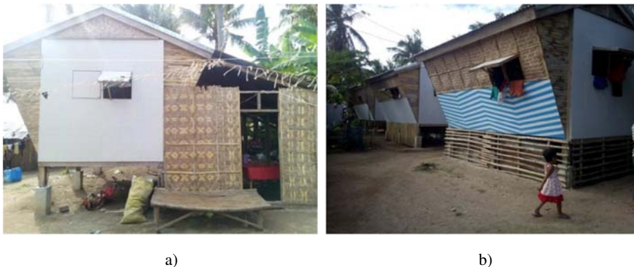
Fig. 8. The inclined roof allowed for an extended overhang, a) for various family activities and the ample space below the shelter, b) became storage for various farm animals
