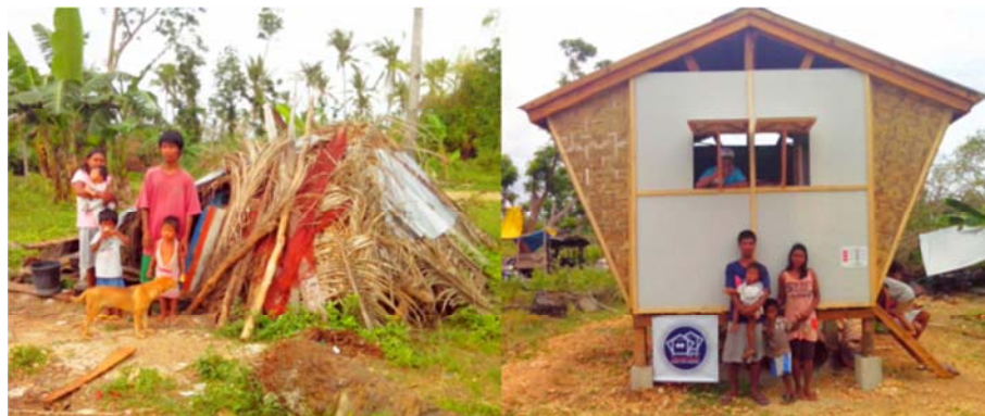
Fig. 7. The first beneficiaries of the transitional shelter through the efforts of Dr. Frtiz Strolz Rotary of Switzerland
