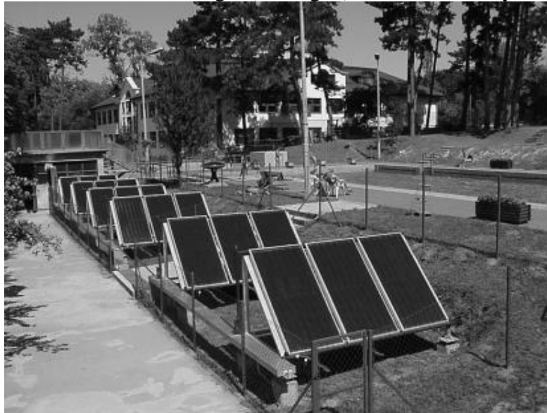
185 Fig. 2. Solar collector field of the measured system 186
