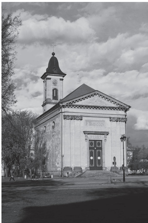
Fig. 6. Heinrich Hatzinger, Julius D'Andreis and Franz Joseph Fohmann: Garrison church in Josefov, 1805–1810 (photo by author, 16 th April 2016)
