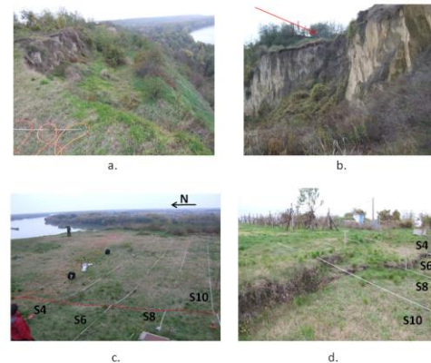
Fig. 3 a. The loess mass which has already slumped looking from the south, (the direction of the study area.) b. The quasi vertical scarp. The arrow indicates the research area. c. The study area from western direction with tapes along profiles S4-S10. The profiles are closely West-East orientated. The dotted red line shows the main fracture which is directly visible from the opposite direction. d. The main fracture from the east with profiles S4-10. The long profile (P2) elongated between two vineyards in line S10.
