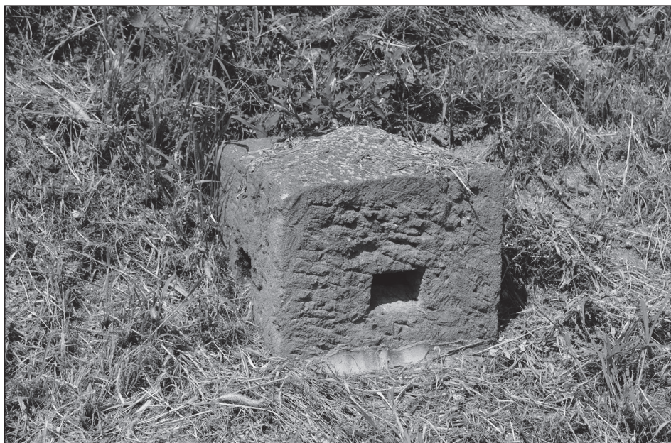
Figure 11. Chimney hatch in the ground surface, 2011. (Photo of Tamás Hajnáczy)
