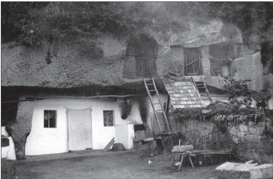
Figure 1. Cave house carved into rhyolite tuff in Sirok (1939) (FORTEPAN: 11485) http://download.fortepan.hu/_photo/download/fortepan_11485.jpg (accessed January 8, 2018.)
