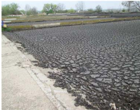
Fig. 7. Sludge fields of WWTP Vráble
