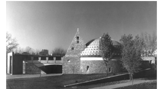
F 07 : Hungary, Budapest-Lágymányos, roman catholic church, 1994-1996. Architect: Ferenc Török and Mihály Balázs (Image by the Architect © Ferenc Török and Mihály Balázs)
