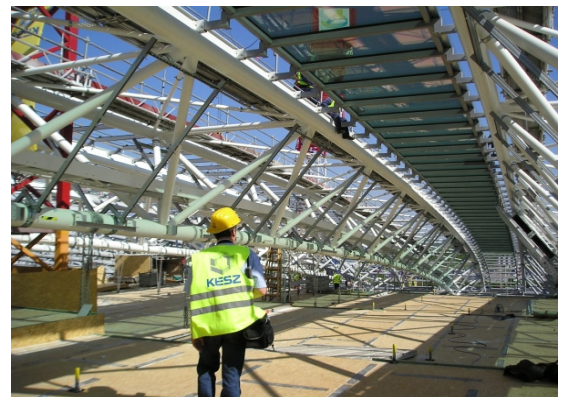
Figure 1. Budapest airport terminal building truss structure
