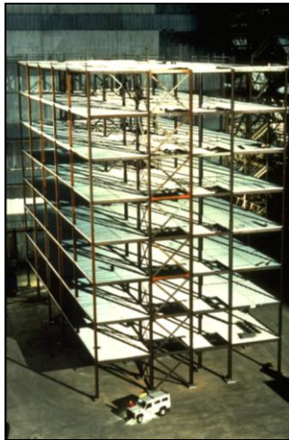
Figure 1.1 Cardington test building prior to concreting of the floors
