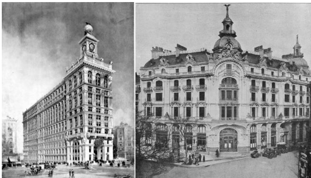
3 (a) New York Life Building in New York City, 1896 (reprod. from: Hudnut 1895, frontispiece) | (b) the second New York Life Building in Paris, 1900 (reprod. from: La construction moderne 16 (1900), pl. 59)
