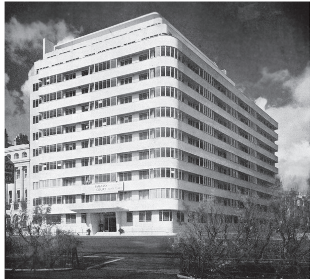
Fig. 44. The Embassy Court in Brighton, architect: Wells Coates (photo published in Tér és Forma 9. 1936. 121)
