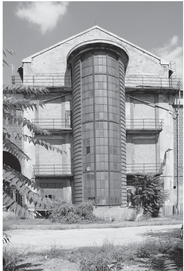
Fig. 15. Kelenföld Power Station, the façade of the 30 kV switch room facing the Danube, architects: Kálmán Reichl and Virgil Bierbauer, 1913/1927–1933 (photo: Galacánu Efstatia, 2008)
