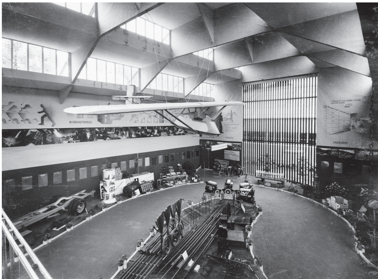
Fig. 52. Interior of the Pavilion of the Rimamurány–Salgótarján Ironworks at the Budapest International Fair, architect: Virgil Bierbauer, 1939; the montage decoration on the wall by Mrs Elemér Marsovszky (photo: MÉM Borbíró-hagyaték GYN: 659. 22. doboz)
