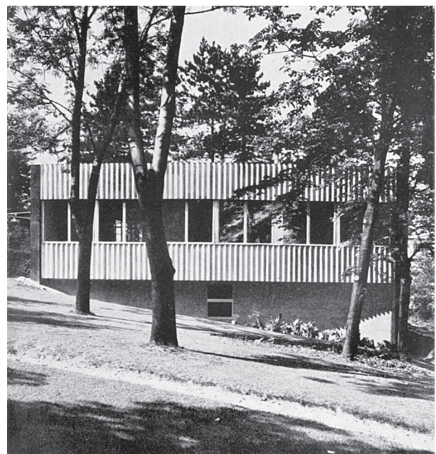
Fig. 24. Family house covered with eternit corrugated board in Budapest, architect: Farkas Molnár (photo: Mrs Elemér Marsovszky; published in Tér és Forma 10. 1937. 372)
