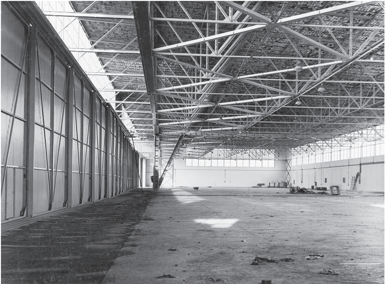
Fig. 31. The interior of Budaörs Airport's large hangar (photo: Zoltán Siedner, 1937; MÉM)
