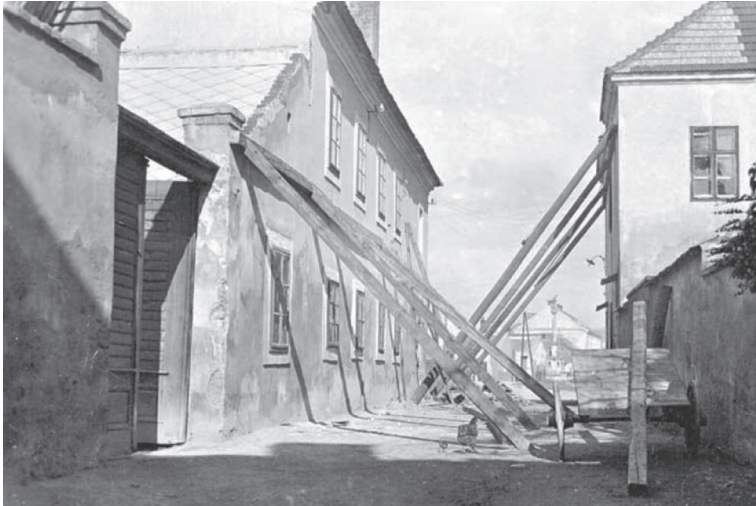
Fig. 6 The picture shows, as an example, houses in Schwadorf in the Vienna Basin supported by wooden struts after the earthquake of October 8th, 1927. The Schwadorf earthquake had a similar epicentral intensity like the 1670 quake in Hall in Tirol. Photo: Archive ZAMG
