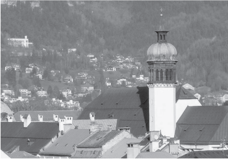
Fig. 8 During the restoration work of the Innsbrucker Hofkirche the globe-shaped decoration at the steeple was analysed. Six contemporary texts were found, five texts reported about the earthquake of December 22nd, 1689 in Innsbruck. Municipal archive Innsbruck. Photo: Ch. Hammerl
