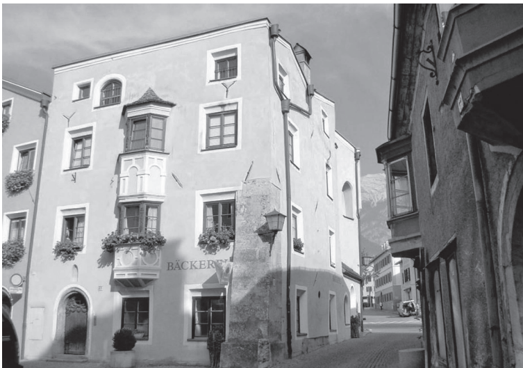
Fig. 5 Probably the heavy damage to the house Agramsgasse 23 was a secondary effect, caused by the partial collapse of the Frauenturm. Earthquake walls, buttresses made of Höttinger breccia were erected and the walls were hold together with iron cramps after the quake. Photo: Ch. Hammerl
