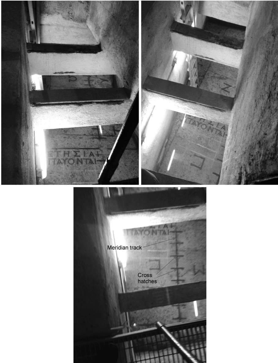
Fig. 6 Views of the track of the meridian and the cross hatches from the catwalk; note reflections of tube neon lamps in the water
