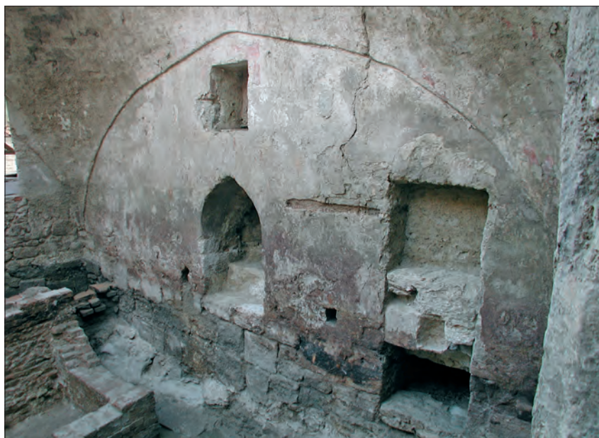
Figure 121. The line of the excavated interior walls of the Esztergom thermal baths (17 th century)
