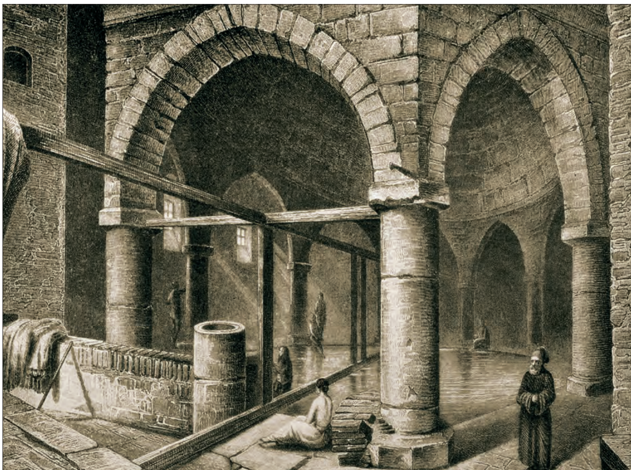
Figure 1. The hot room of the Rudas Baths in Buda in an engraving by Ludwig Rohbock, 1859
