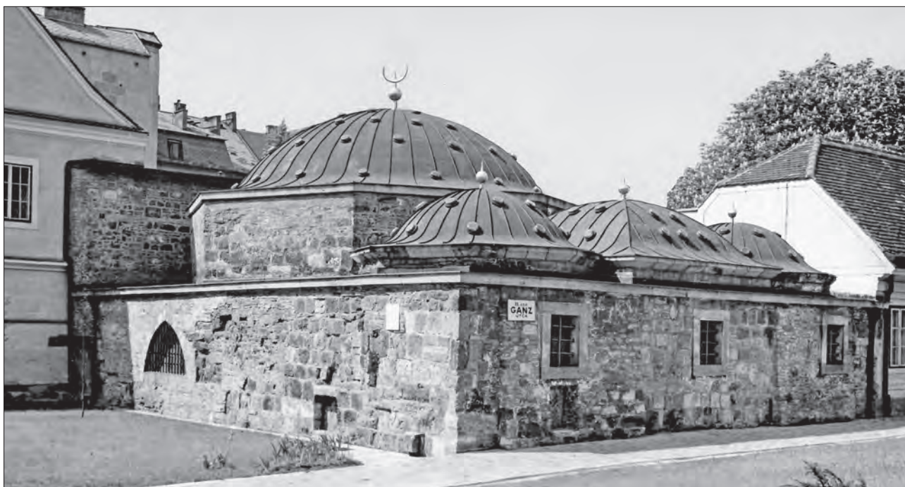
Figure 102. The Király Baths in the 1960s, following refurbishment
