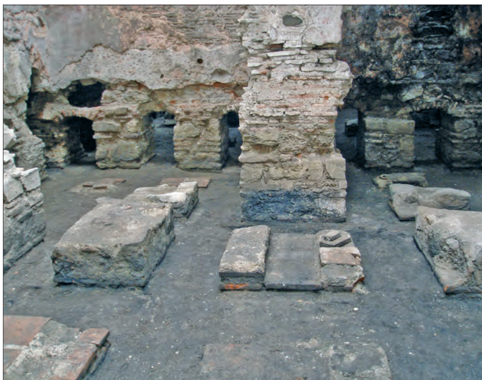
Figure 63. 14 th -century columns excavated at the Murad I Baths in Iznik that were part of the underfloor heating system
