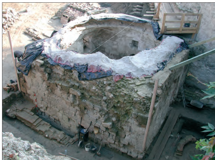
Figure 122. Exterior of the excavated 17 th -century thermal baths in Esztergom
