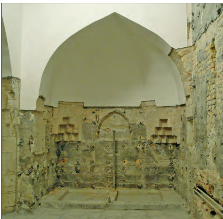
Figure 91. The Császár Baths hot area, iwans located on the south side, during excavations
