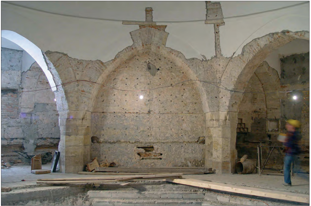
Figure 90. The Császár Baths during the excavation of the hot room
