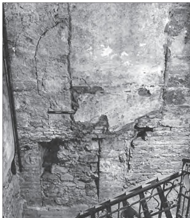
Figure 103. Ottoman era window uncovered during restoration work at the Király Baths
