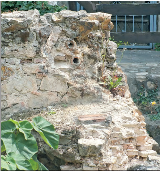
Figure 111. The water pipes visible in the wall of the double baths at Székesfehérvár
