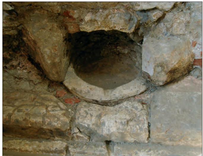
Figure 54. A well sunk beneath a stairway in the excavated entrance hall of the Rác Baths, photographed from above
