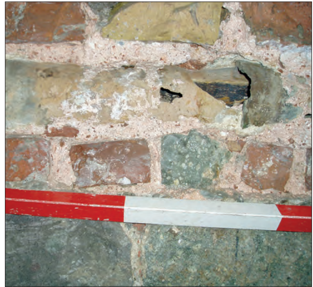
Figure 62. Ottoman era ceramic waterpipes excavated from the wall at the Rudas Baths
