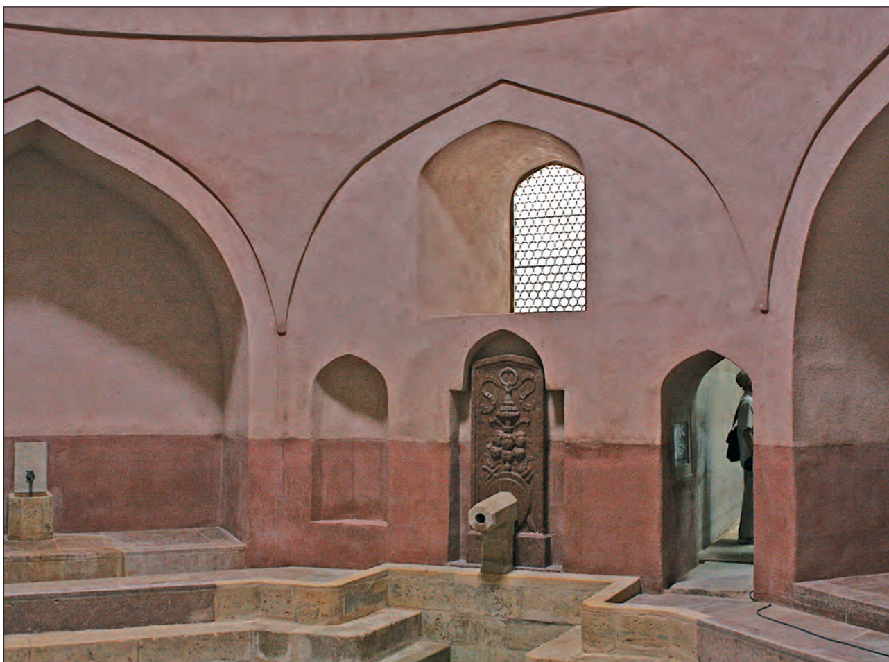
Figure 94. The hot room of the Rác Baths following restoration
