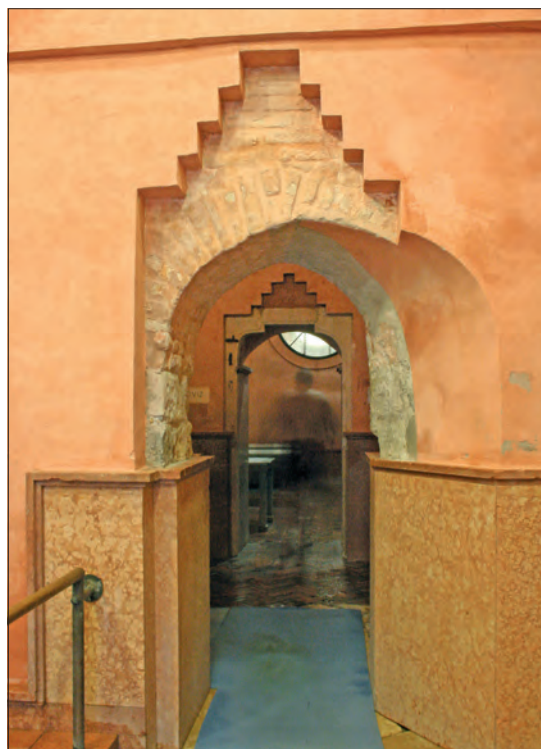
Figure 82. Stepped ornamentation of the doorway between the warm rooms at the Rudas Baths following reconstruction
