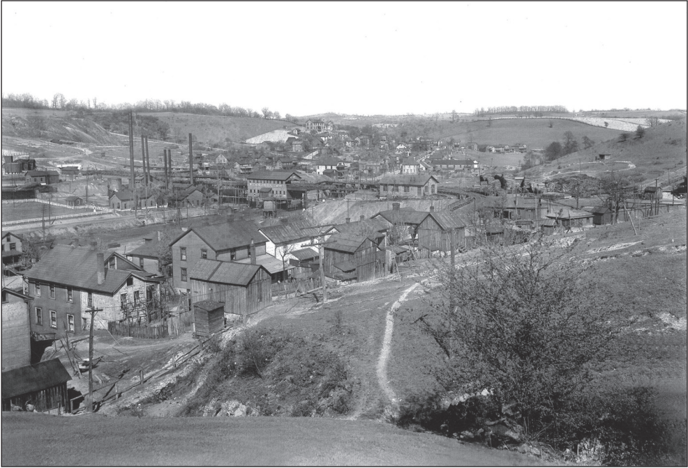
Figure 1. Westmoreland Mining Company's Mine #2. Pennsylvania, 1918. Photo by John Sartoris
