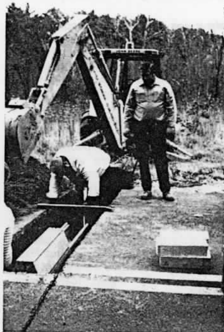
Workmen installing the tunnel at Amherst. (PHOTO: D. Pierson)
