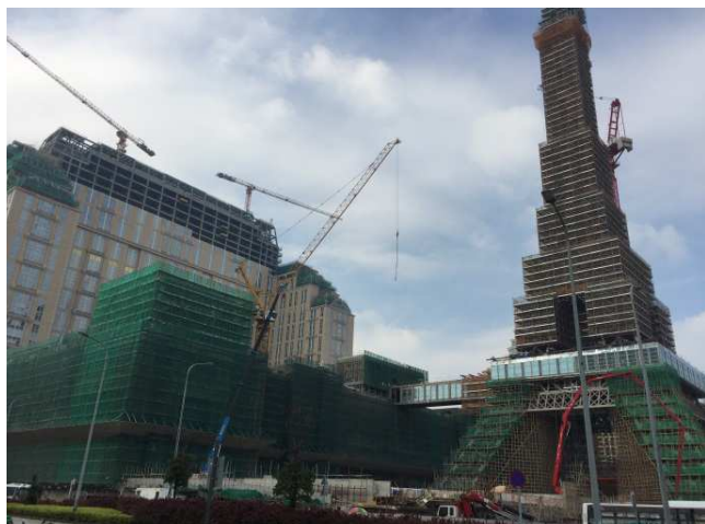
“Paris” under construction
