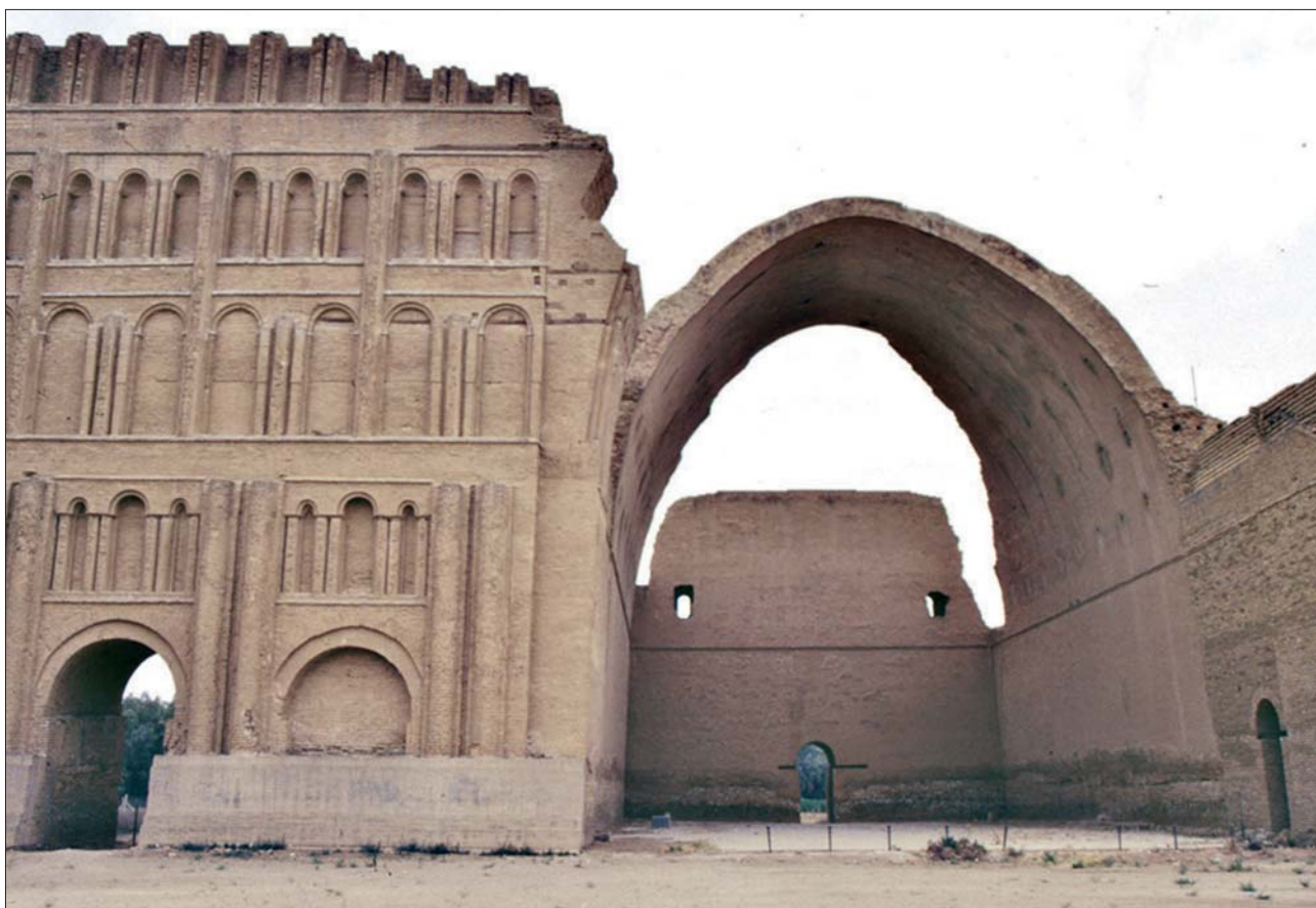
Fig. 20. Tāq-i Kisrā (today in Iraq): the single still extant architectural remain, probably the one-time throne room, of the palace of the Persian ruler in Ctesiphon
