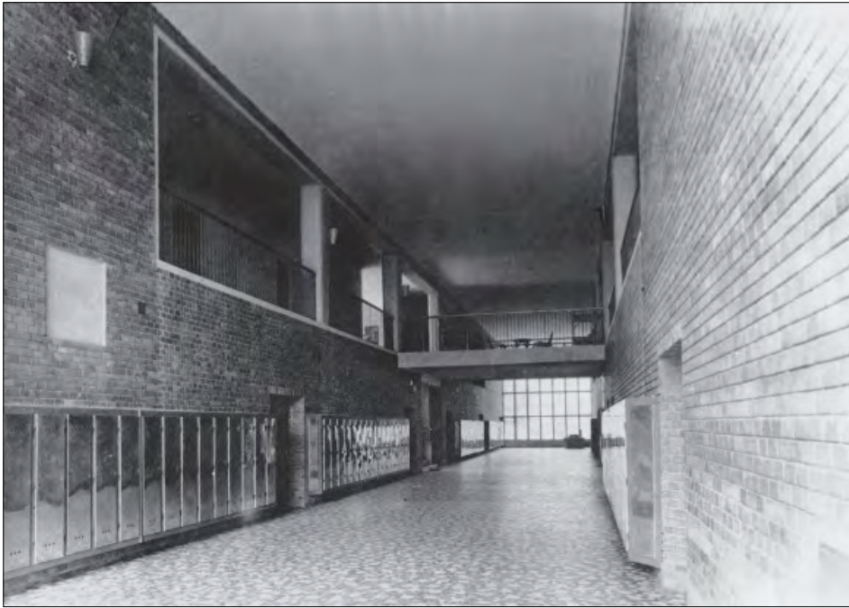
Figure 1. Kismarty-Lechner Kamill Kismarty-Lechner: Primary school in Budapest, Sodronyos st. 1955–1958. [2]
