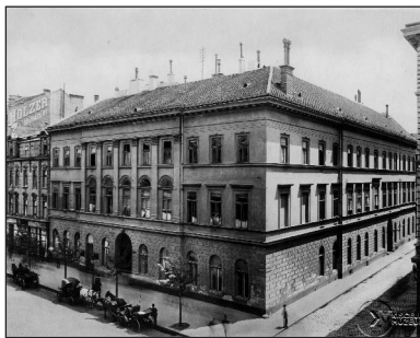
1. Figure The building of the National Casino
