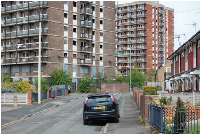
Fig. 3. Manchester, buildings before their demolition in Islington, 2013 (Photo by the author)
