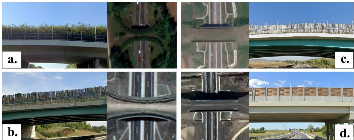
Figure 4 The noise barrier/screening design variations (a.: vegetation only, b.: wood pile and vegetation, c.: wood pile only, d.: panels)
