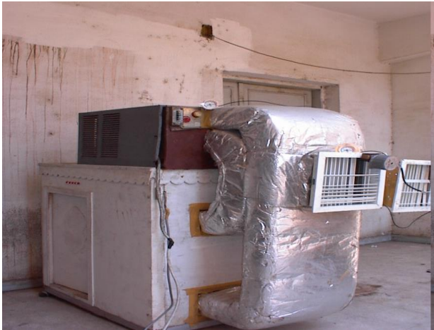
Figure 2: Photo for the proposed test section
