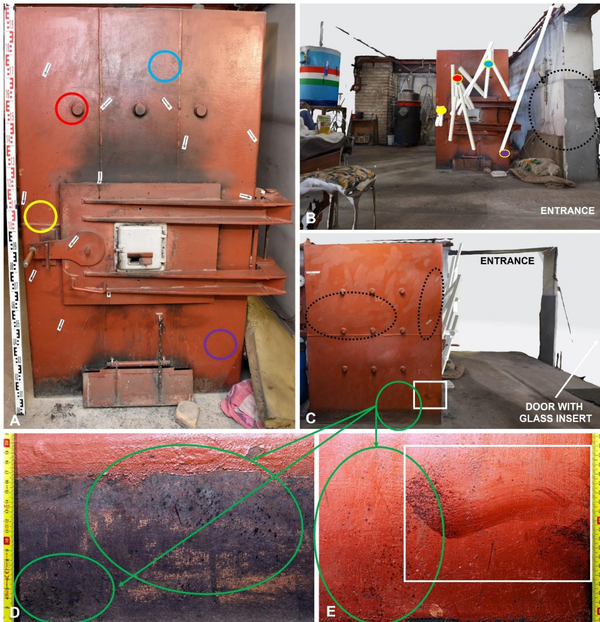
Picture 1: The boiler with blood stains 14
