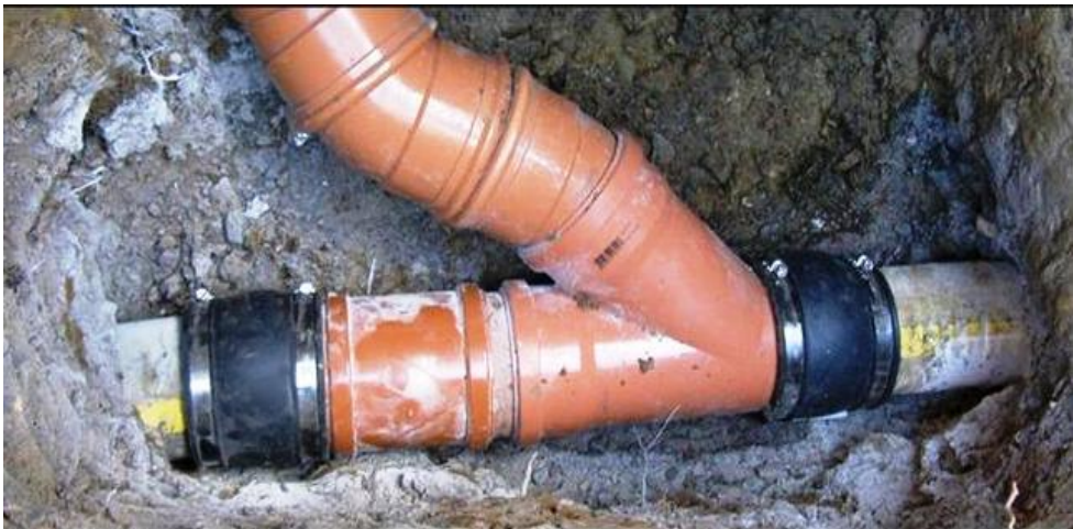
Photo 5: Sewage pipe repair. Source: 21
