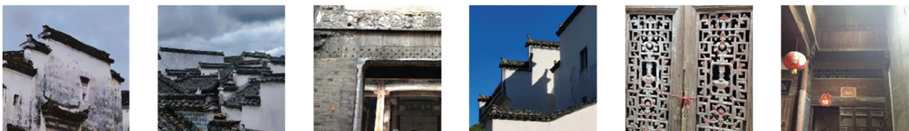
Fig. 6. White wall, Black tile, Gray brick, Horse head wall, Lattice window, Wooden element (Photo: Author)
