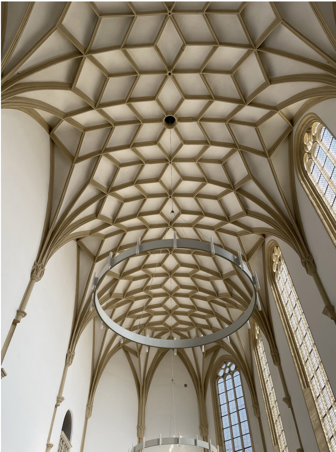
Figure 2. The vault of the Reformed Church of Nyírbátor
