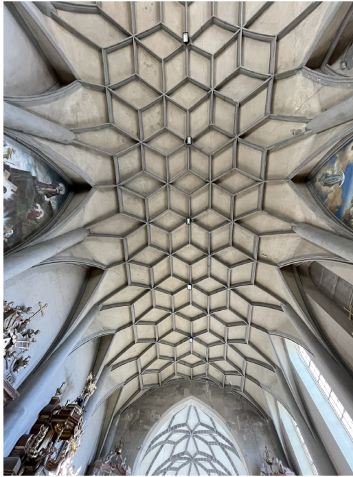
Figure 1. The nave vault of the Franciscan Church of Szeged-Alsóváros
