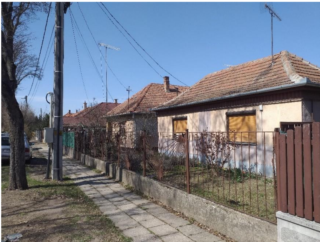
Figure 30. Houses from the 1960s in the garden city zone (Debrecen, Hungary) (Photo taken by the author)
