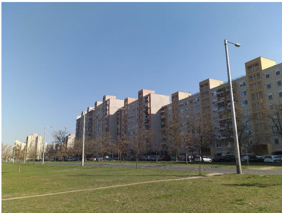
Figure 34. Housing estate from the mid-80's (Debrecen, Hungary) (Photo taken by the author)
