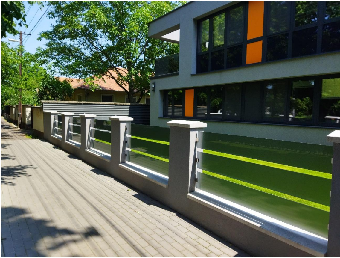
Figure 56. Fence built according to CPTED principles (Debrecen, Hungary) (Photo taken by the author)
