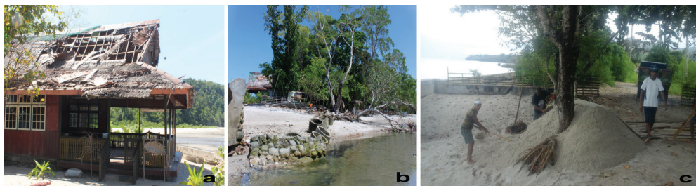
Figure 9. a – Kewang house was broken, b – the occurrence of abrasion, c – local people transport sand from other locations to be relocated in the beach (Photo by: H. G. Saiya)
