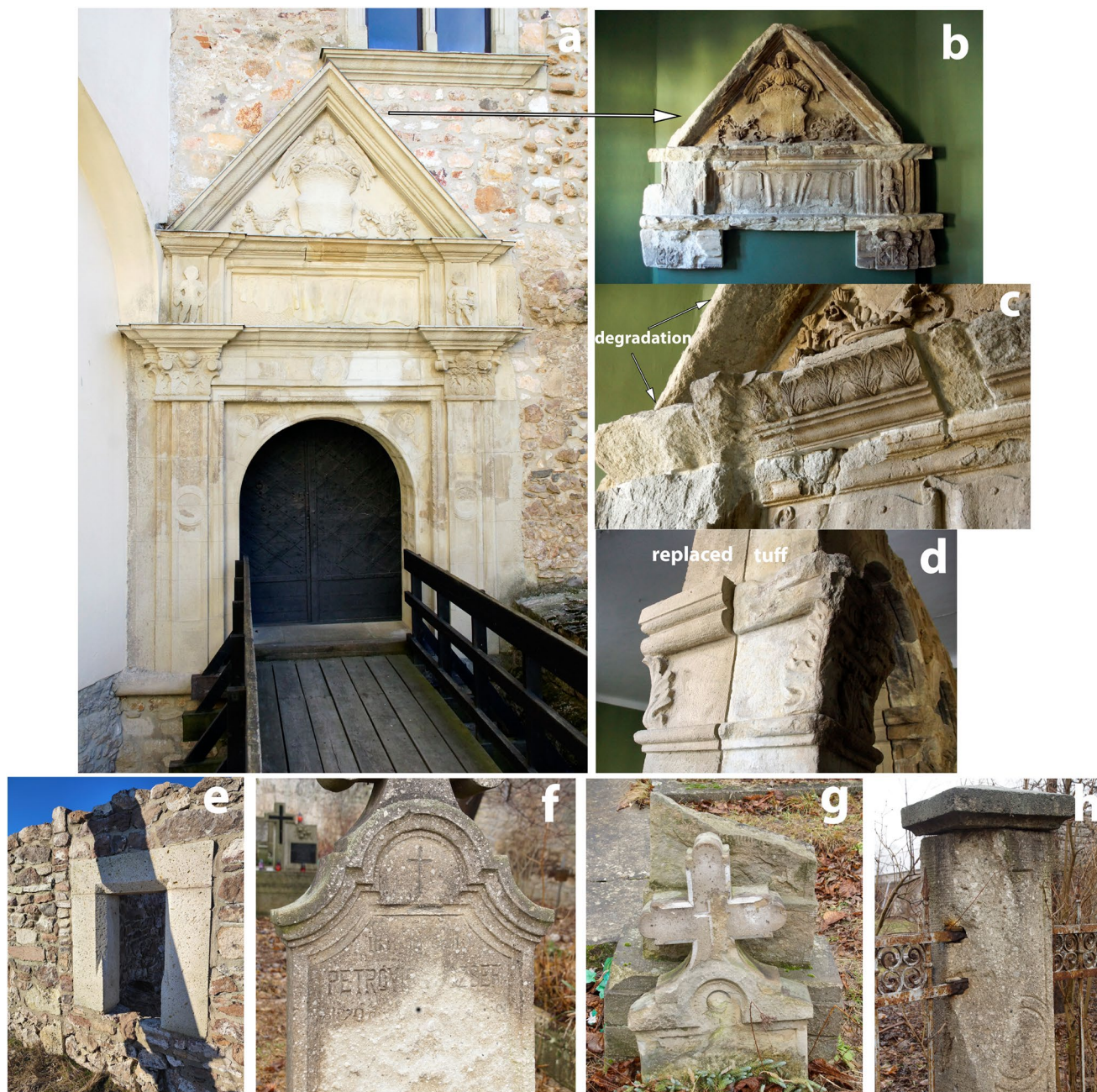
Fig. 7 Degradation of decorative stones. Vágáshuta Tuff : (a) Large gate of Red Tower (Sárospatak Castle) replaced by artificial material. (b-c) Original degraded stones of the gate in the museum. (d) Unique combination of original and artificial stone showing the difference in
