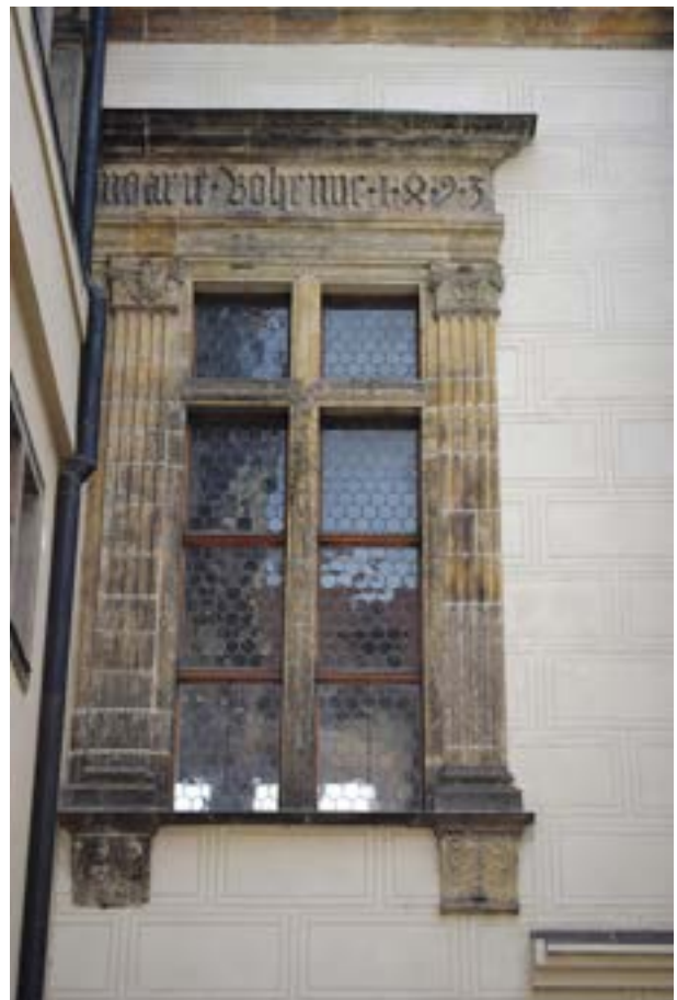
Fig. 26. Window of the courtyard façade of the Great Hall of the Vladislav Wing in Prague Castle, 1493
