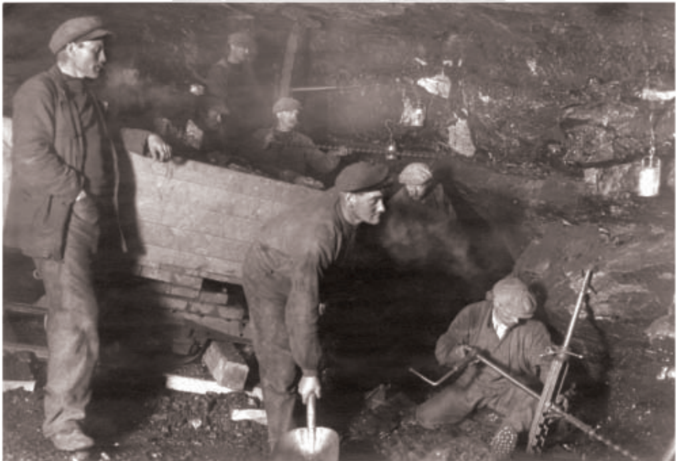
Coalmining at Svalbard. Minors at work down in the mine. Coal is being loaded on to the railway cars. Photo: Sigvald Moa, 1918, Svalbard (Norway)
