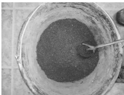
Figure 3 Mixing cement and perlite
