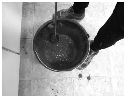
Figure 4 Fresh cement slurry after mixing
