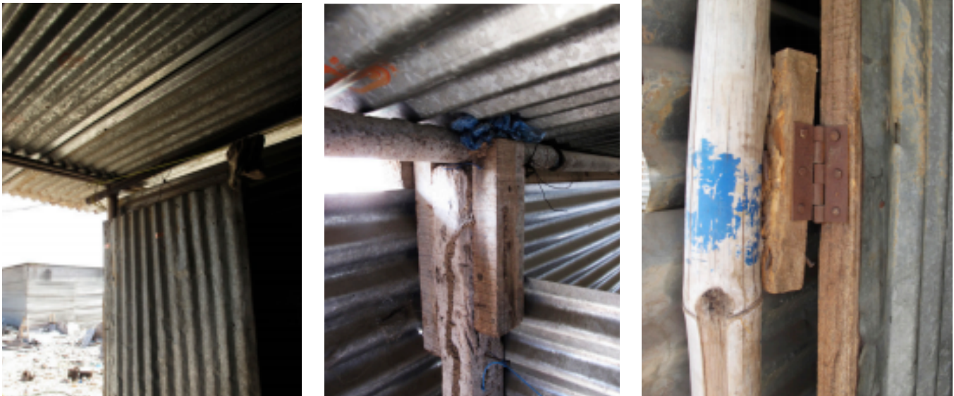
Figure 15. Use of commonly available materials and impromptu joinery details.
