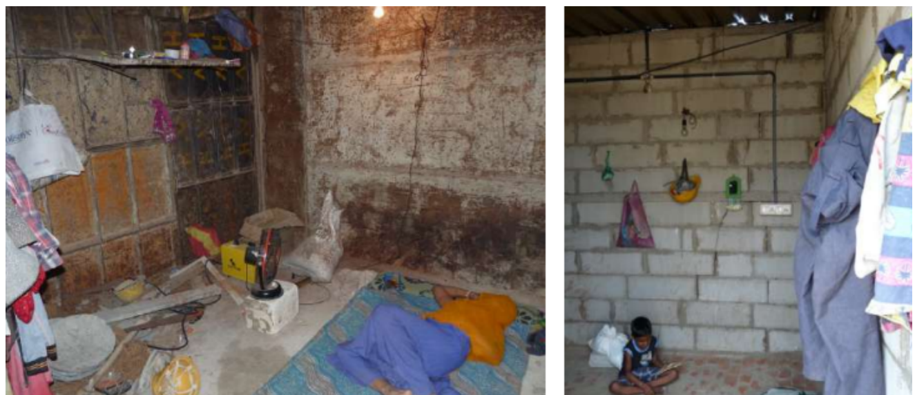
Figure 11. Hanging electrical wires to make arrangements for a bulb, extension board and fan.
