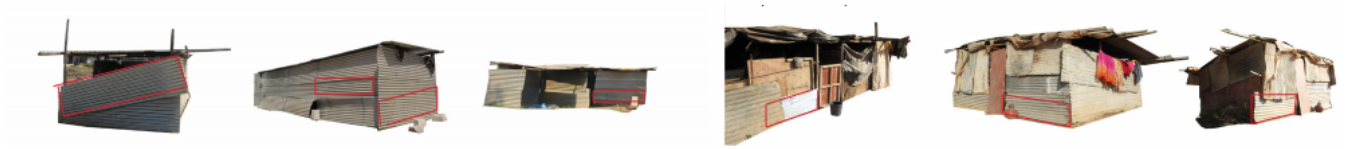
Figure 14. The image displays a 800 mm X 2030 mm corrugated sheet commonly used for the worker housing.
