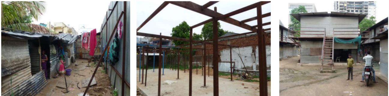
Figure 5. Frame structure made by fabrication onto which corrugated metal sheets are bolted, also a single storied structure is seen built with the same assembly.
