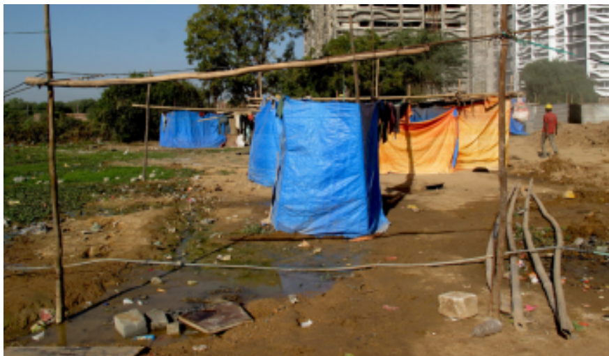
Figure 16. The toilet areas covered with tarpaulin sheets with improper drainage left to run along the site peripheries.
