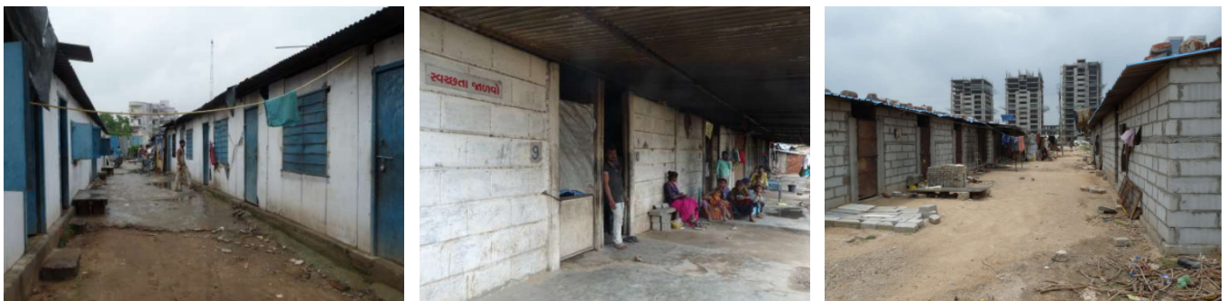
Figure 6, 7, 8. Rooms made from Aerocon panels (Aerocon sheets are cement sandwich panels, made of two fibre reinforced cement facing sheets on either side of a light-weight concrete core).
