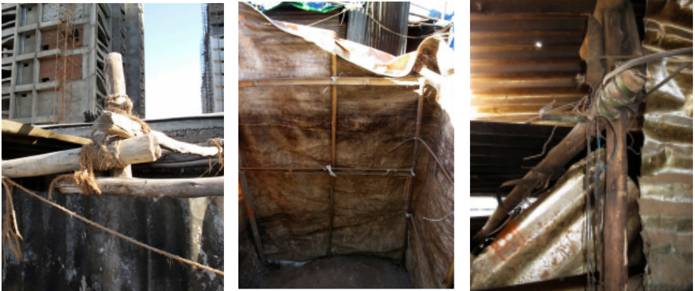
Figure 17. Use of commonly available materials and impromptu joinery details.
