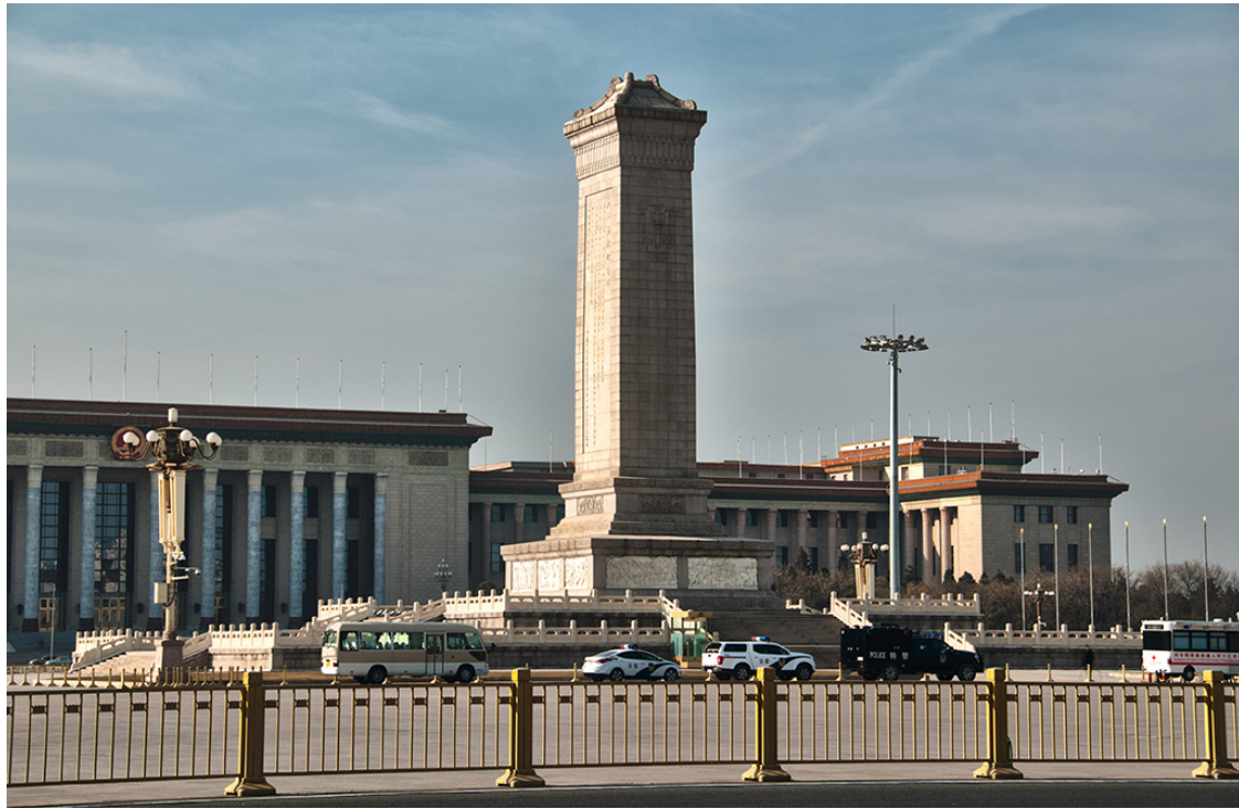
Figure 2. The Monument to the People's Heroes at Tiananmen Square, Beijing. Note the presence of a Chinese-style curved roof instead of a traditional pyramidion. Source: C. Langer, January 2019.
