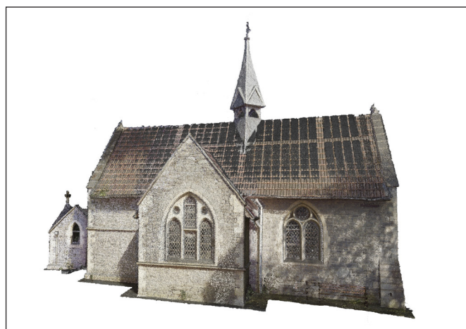
Fig. 10. Point cloud of the chapel of the Feriköy Protestant cemetery created with a TLS scanner (Made by: Gergő Máté Kovács, 2021)
