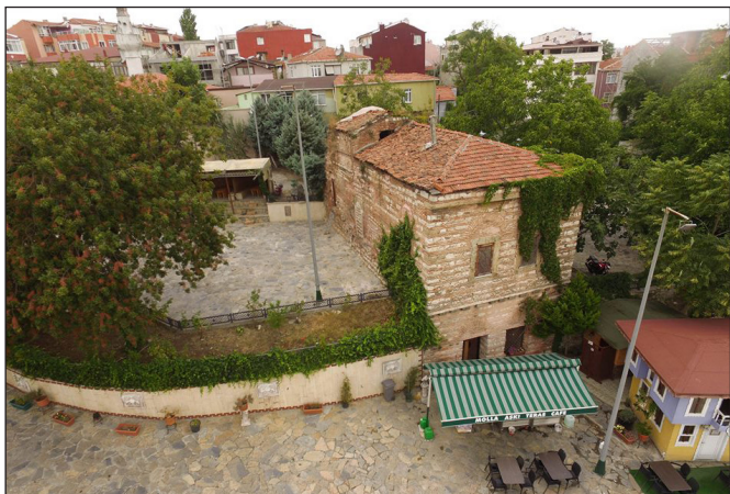
Fig. 2. The house of the Transylvanian Ambassadors in Istanbul, distant view (Photo: István Pi Tóth)
