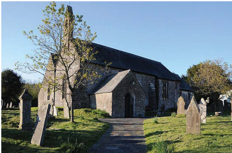
Figure 3. St. Michael’s Church, Myddfai. Burial place of descendants of the “Physicians of Myddfai.” (Philip Halling Å, source: https://commons.wikimedia.org/wiki/File:Myddfai_church.jpg )
