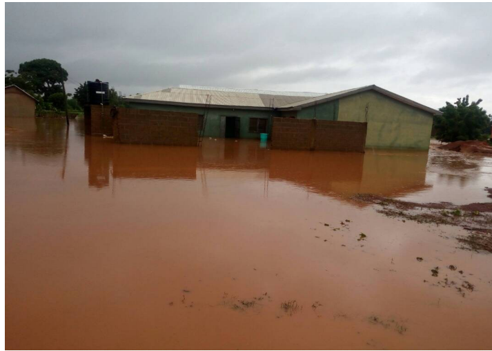
Figure 4. Compound Inundated by Floodwaters in Tamale
