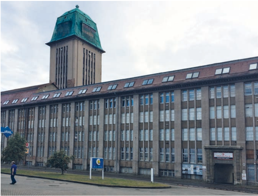
Figure 2. Former factory building of the company Ludwig Hupfeld AG in Böhmlitz-Ehrenberg, Leipzig (photo: Andreas Meyer)
